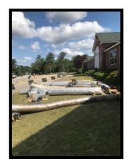
Even with the school closed, there are great things happening on "The Hill." Our Encapsulation project is well underway. TSA parent, Michael Laney and his team, are removing the ducting, replacing HVAC with split units, and creating a more energy efficient and cleaner air and heating for our elementary classrooms.
